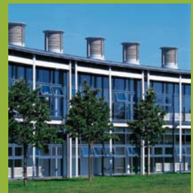
Haute Vallee School Theatre, Jersey
